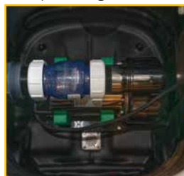
Check valve and sewage pump Mach II
