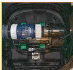
Check valve and sewage pump Mach II
